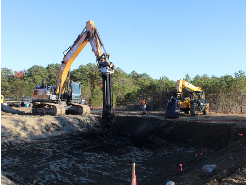
In situ soil mixing of carbon and calcium additives
